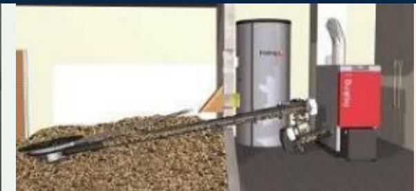
Interior Silo holds 12 tons of Dried wood chips
