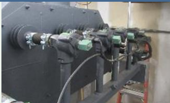
Viessmann Pyrot 540 KW boiler has 1,843,000 BTU/hr peak output Features: Flue gas recirculation, Pneumatic tube cleaning
