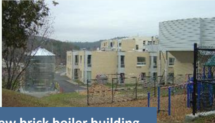
New brick boiler building matches school
