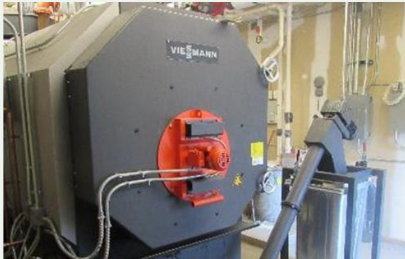
Viessmann Pyrot 540 KW boiler has 1,843,000 BTU/hr peak output Features: Flue gas recirculation, Pneumatic tube cleaning
