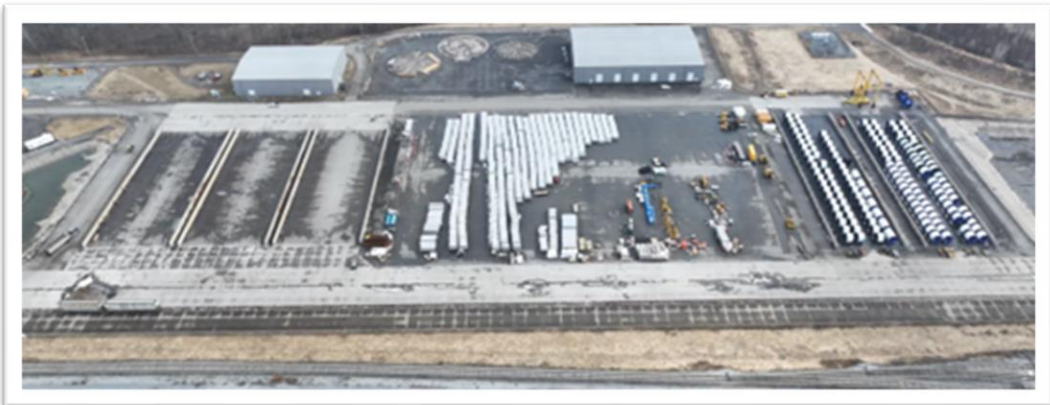
Fort Edward Laydown Yard
