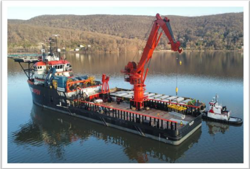
Concrete Mat Installation – Hudson River
