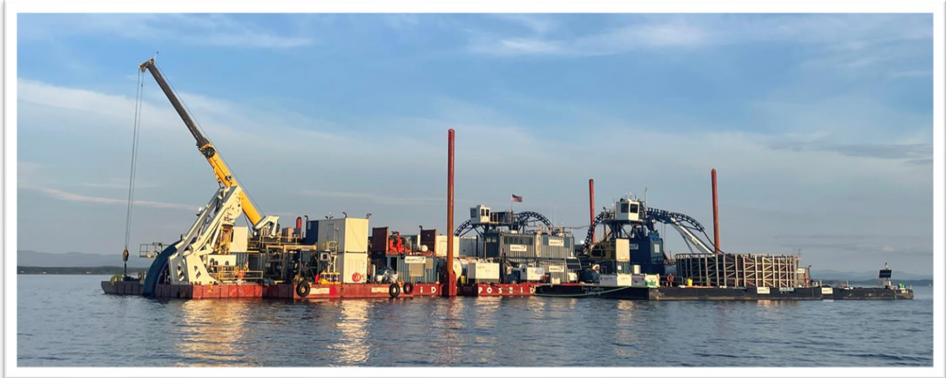
Cable Installation Barge – Lake Champlain
