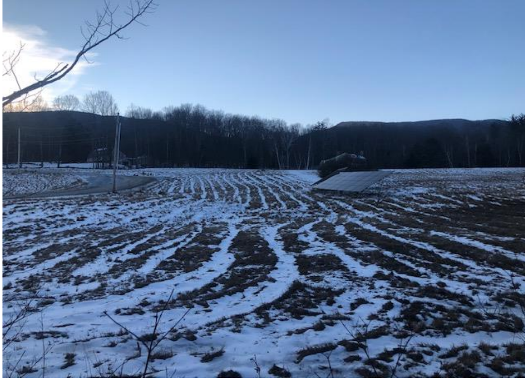
22.5kW AC residential solar array
